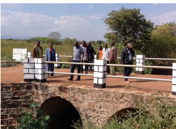
a) Rehabilitated bridge
