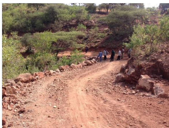
b) Rehabilitated feeder road
