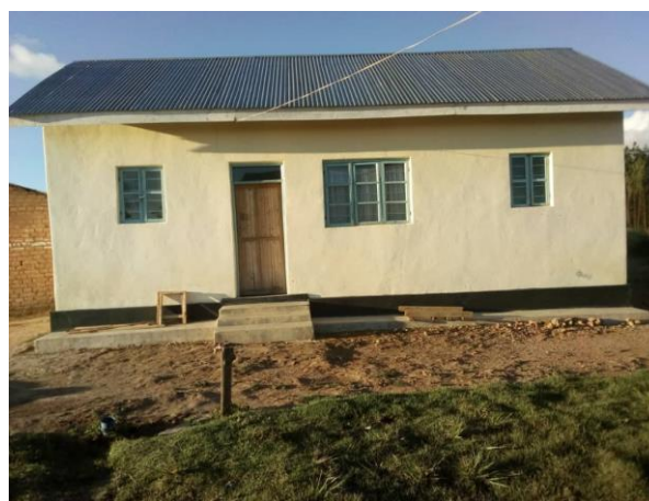
Community constructed nurse's house
