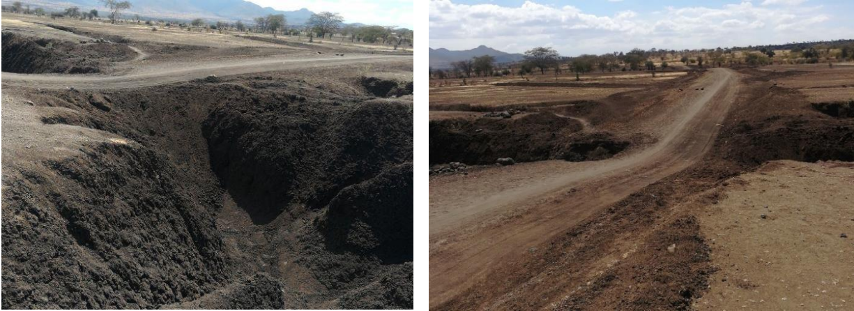
Plate 3: Constructed Road in Losimingori Village in Monduli
